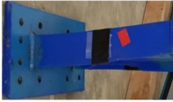
Fig. 8. Damage on WRBSC beam flange.
